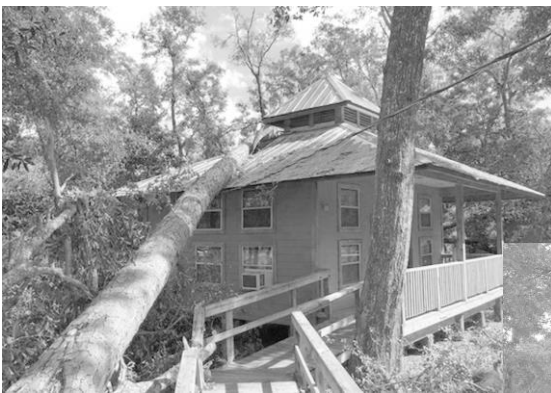
Damage to Camp Dogwood Acres structures as a result of Hurricane Michael in Panama City, Florida.
